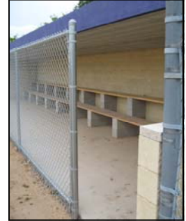
Newly renovated dugouts at McCarty Field.
