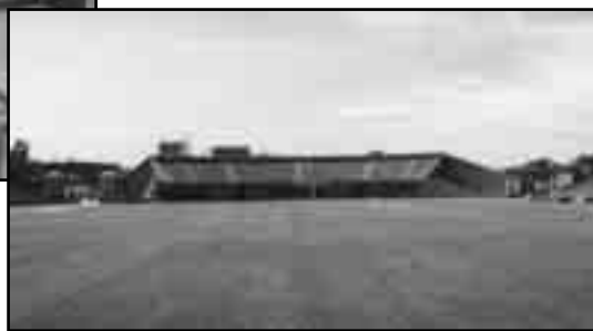
New stadium additions and football offices
